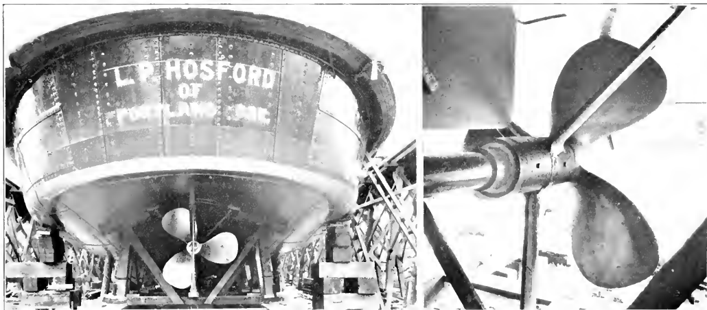
Two views of the stern of the L. P. Hosford on the ways in the builder's yard showing lines of tunneling and arrangement of rudders and outboard propeller shaft bearings.
